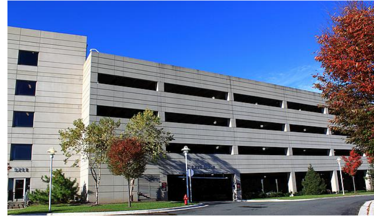
Multi-level parking garage
