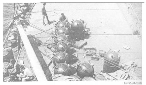
Contact mines on board the captured Iranian minelaying ship Iran Ajr.
