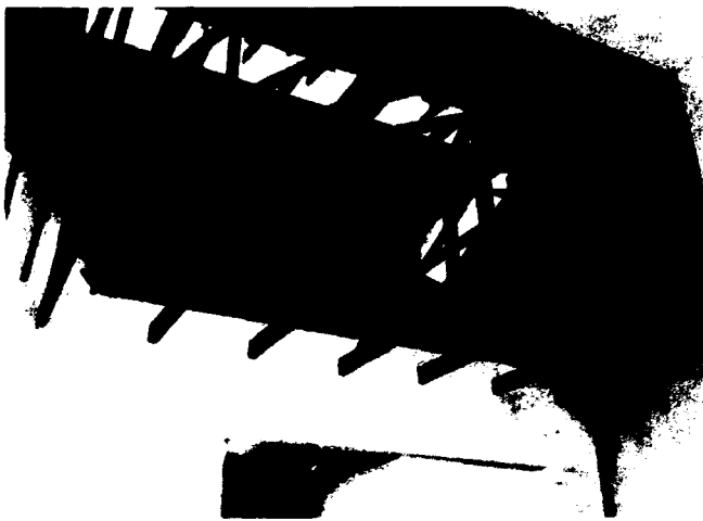
FIG. 70. OLD AND NEW RAFTERS WEAVING: Weatherbee, Hailey. Uxbridge Ontario, 2013.
