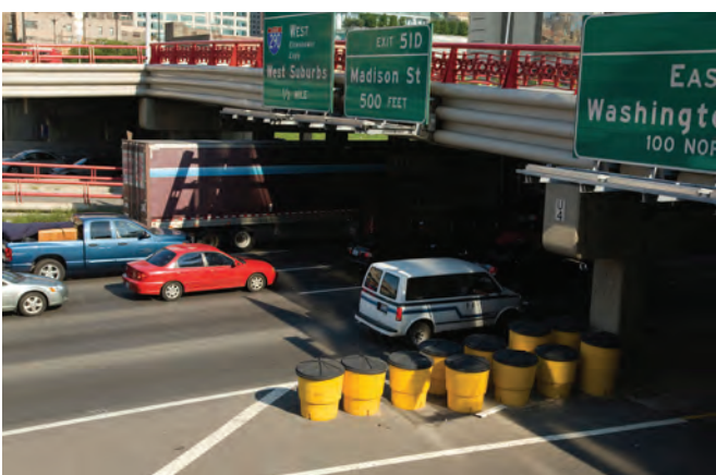
Figure 5.12 A car would lose a lot of its energy hitting the barrels. It would be a lot less damaged than if it hit the pillar directly.
