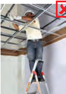
Wrong standing position
