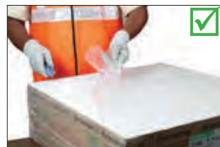
Step 2: Remove the polythene film
