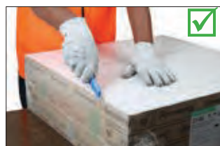
Step 1: Cut the polythene film
