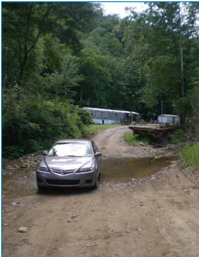
Figure 3.3-1. Low water crossing - this can be suitable for very low-volume access. Unimproved ford is a natural crossing that is undesirable for daily use.
