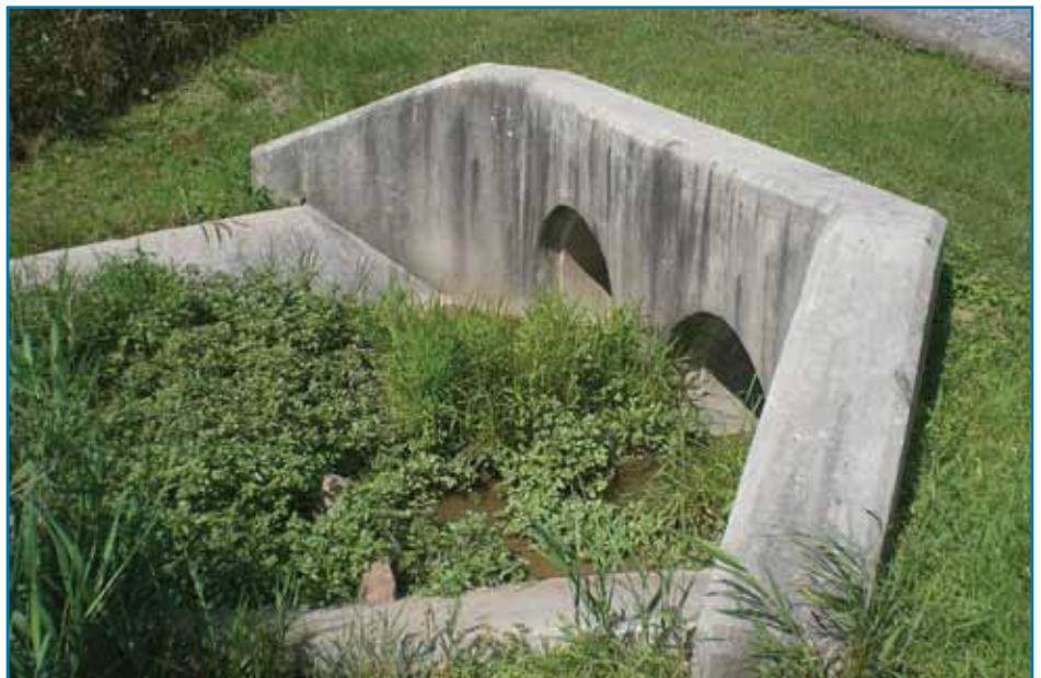
Figure 3.2-5. Multiple culverts at driveway ditch crossing have adequate spacing and compaction. The concrete headwall and wing walls help direct water flow and prevent washouts during high water flow. There is also adequate cover and culvert length to allow liberal clearance of traffic.
