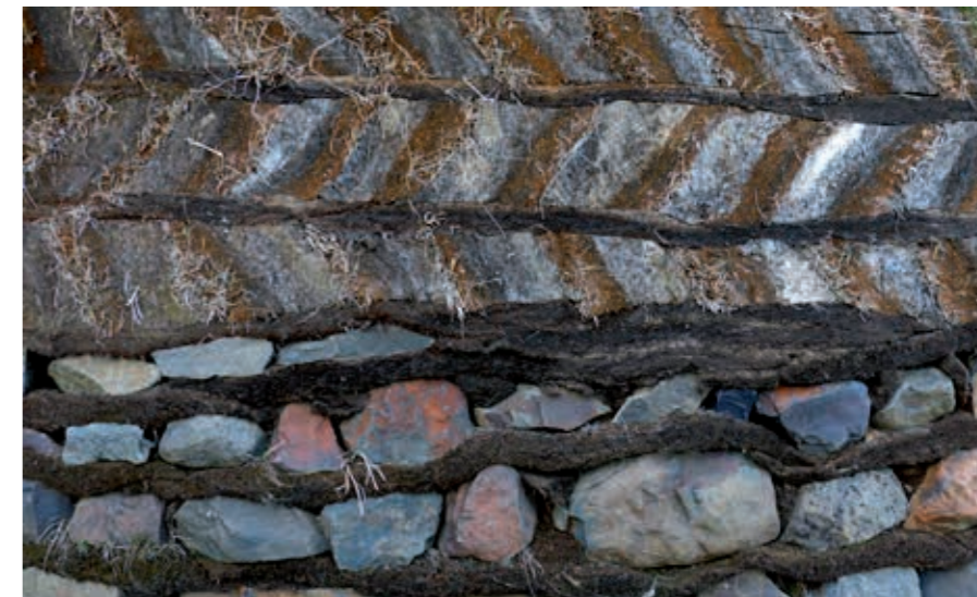
Above: A common way of using turf was to cut blocks from clay-rich ground using a spade, and lay them in courses to form a thick wall. The plant roots bind the earth blocks together and a wall can be erected quite quickly. Turf was also laid in courses between stones to form masonry walls without mortar.
