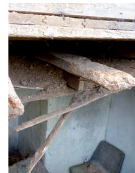
Below: clay deafening between floors, Horn.
