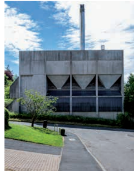
Dingleton Boiler House in Melrose (1977).
