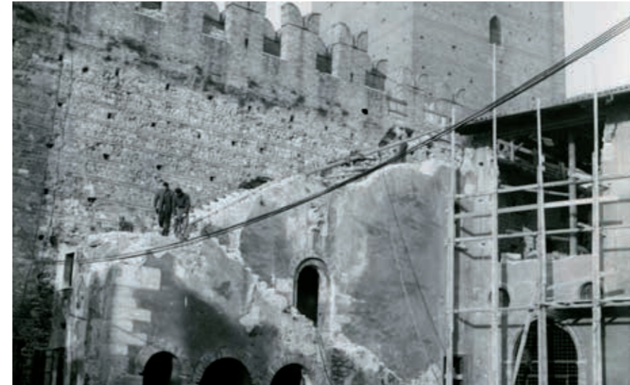
Simultaneous demolition of façade and staircase to create space for the Cangrande statue. © Castelvecchio Museum archive
