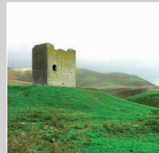
Dryhope Tower Scottish Borders
