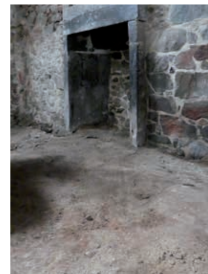
Below: a clay floor, Longforgan.
