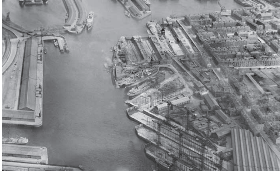
Yorkhill Quay and Harland and Wolff Shipbuilding Yard, Clydebrae Street, Glasgow: aerial photograph taken facing the south-east dated 1931. © HES (Aerofilms Collection)
