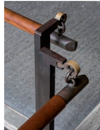
Detail of handrail in gallery. © Peter Guthrie
