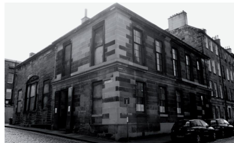
Above: The Glasite Meeting House on the corner of Albany Lane and Barony Street. 'Glasite Meeting Hall 01' by byronv2 licensed under CC BY-NC 2.0.
