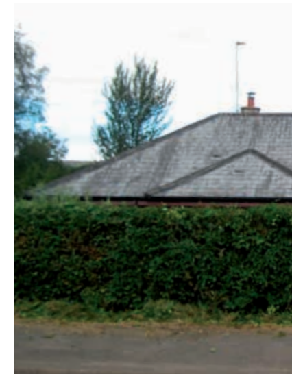
Artificial concrete tiles. All images © Patricia Woodley except where stated otherwise.
