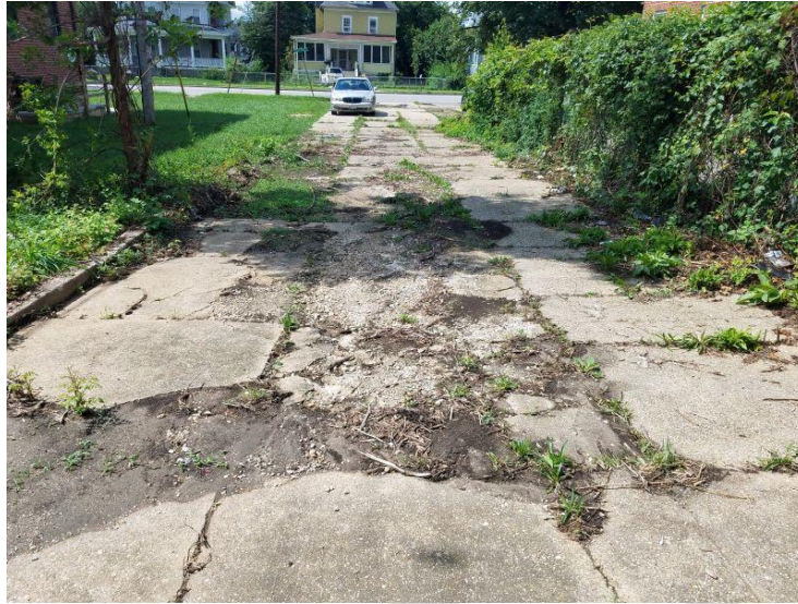
Image above: Current conditions at Fordney Lane.
