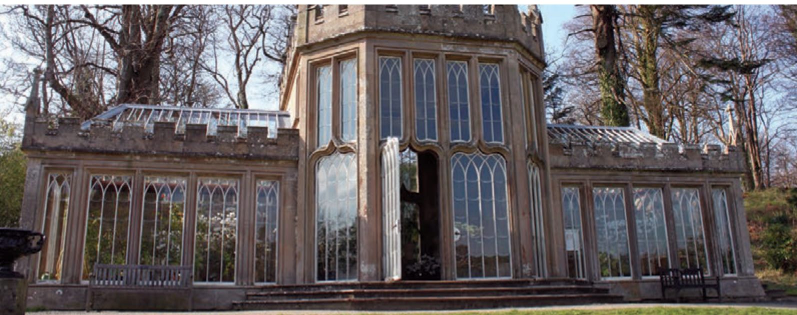
The category A-listed Camellia House at Culzean. © Crown Copyright
