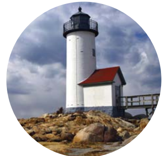
ANNISQUAM HARBOR LIGHT STATION, GLOUCESTER
