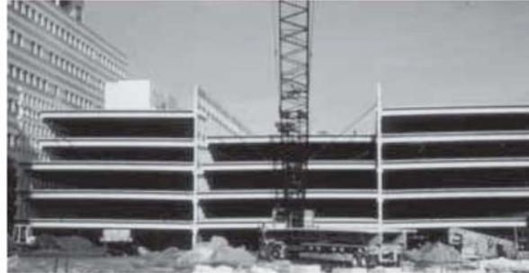
Figure 7-1 Crane in middle bay setting three bays at a time – bringing the building out in one sequence.
