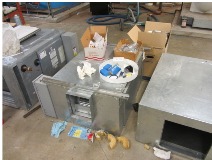
2: Typical Water Source Heat Pump
