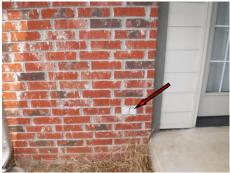
• Repair: Damaged outlet cover plate should be replaced to avoid a shock hazard. Attic and Garage.
