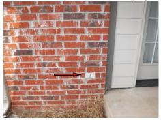
• **Repair:** Damaged outlet cover should be replaced to avoid a shock hazard and water damage to the outlet. *Exterior* (back of house).
