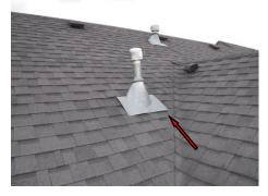
• Monitor: The flashing is vulnerable, has leaked in the past, and should be watched carefully for leaks.
