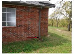
• **Repair:** The gutters require cleaning to avoid spilling roof runoff around the building – a potential source of water entry or water damage.
