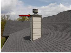
• **Repair:** The paint on the trim around the siding is peeling. These areas should be painted to prevent water damage and rot. *Fireplace Chimney Chase*.
