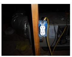
• Repair: An outlet is damaged. It should be replaced. Pantry. Marked with an orange sticker with a "D".
