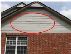
• Repair: The siding trim needs caulking improvements in localized areas to prevent water damage and rot. See Pictures.
