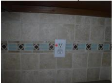
• **Repair:** The installation of a ground fault circuit interrupter (GFCI) is recommended. A GFCI offers increased protection from shock or electrocution. *Exterior* (all).
