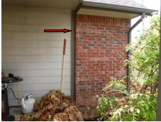
• Repair: Localized rot was observed in the trim around the siding. Fireplace Chimney Chase.
