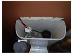
• Repair: The toilet runs on after flushing. Improvement to the tank mechanism is likely to be needed. Guest Bathroom.
