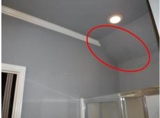
• **Monitor:** Typical drywall and/or plaster flaws were observed that could include loose tape, minor cracks, rough seams, peeling paper, nail popping, minor patching, loose or bulging plaster, etc. Any repairs would be discretionary.
