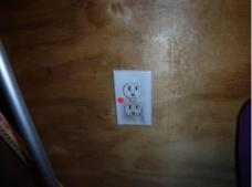
• **Repair:** An outlet is loose. It should be repaired. *Kitchen. Marked with an orange sticker with an "L"*.
