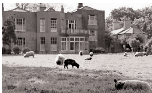
Sheep grazing at the old Clareville (demolished 1988)
