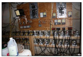
Indoor marijuana grow houses require massive amounts of water and electric. In order to prevent detection, growers redirect the systems that bring these services into the house and tamper with the meters that measure consumption. The cost to cover the higher consumption of electricity and water is passed along to all consumers. Diverting electricity and tampering with electrical wiring can lead to house fires. The use of extra exhaust fans in the grow house can accelerate the
