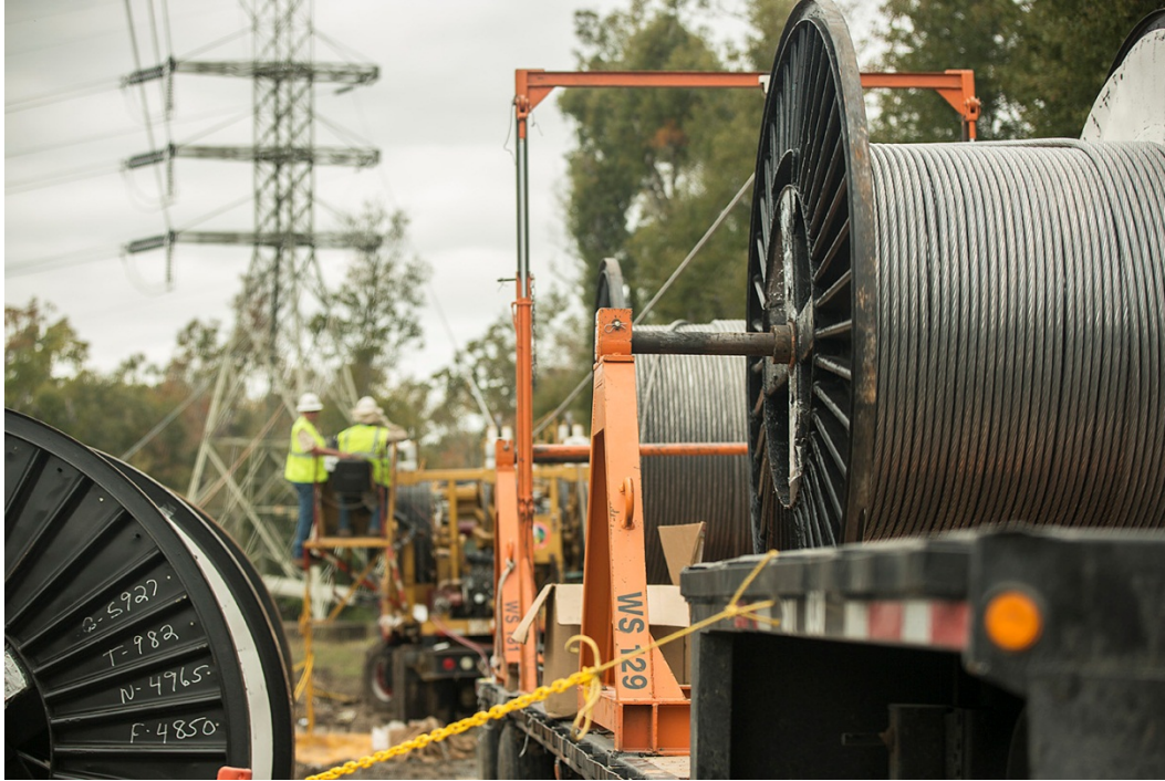
Figure 3: Pulling the conductor to ground to install the traveling ground is commonly done using a single rope. This could kink the conductor if tension was high enough. Use a 20x diameter (51 cm) guide roller, or slacken the conductor if it needs to be lowered to install the traveling ground. Photo courtesy of CenterPoint Energy.
