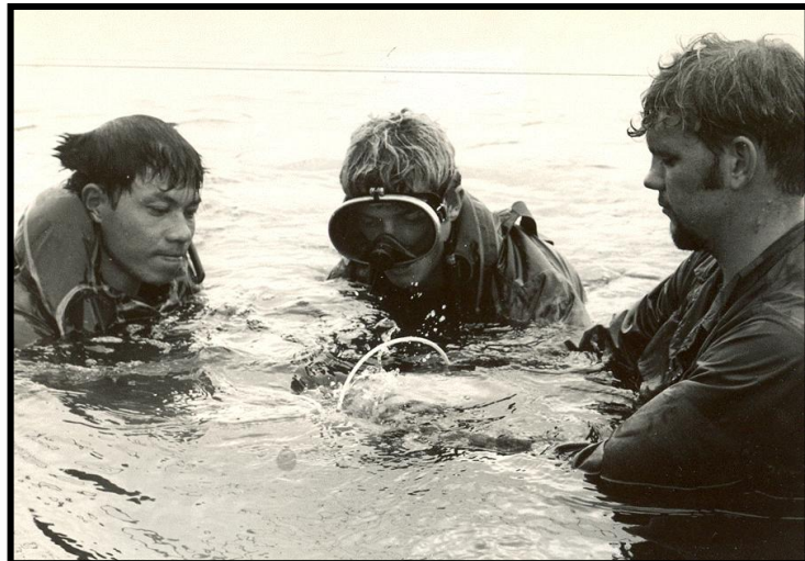
Nam Can Canal, RVN, 1970: Combined US and VN Navy operation in support of Operation SEA FLOAT. This photo shows detonation cord being wrapped to the end of Mk 1 explosive hose. The hose was placed on the river bottom with the cord leading to the surface where it and the blasting cap/time fuze was floated on an air mattress. (photo courtesy of CDR L. E. Ronan, USN, ret.)
