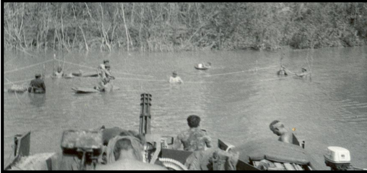
Nam Can canal, 1970: EODTEUPAC Team 82, VNN Underwater Missions Battalion (EOD Company), UDT 13, and SEAL Support personnel explosively deepen a canal connecting “old” Nam Can with “new” Nam Can (a US Navy afloat base named “Sea Float”)—a distance of approximately 20 miles, to allow friendly patrol craft to pursue VC and NVA that had used the area between to two villages as a sanctuary. This area was also an infiltration route for enemy forces. This photo shows explosive hose being offloaded from a Heavy SEAL Support Craft (HSSC) on to air mattresses for further placement on the canal bottom. The connected hose sections were then detonated to provide channel deep enough to allow access by Market Time PBR’s. Several prisoners were taken during this operation. (photo courtesy of CDR L. E. Ronan, USN, ret.)
