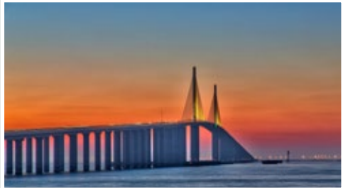
SUNSHINE SKYWAY BRIDGE
