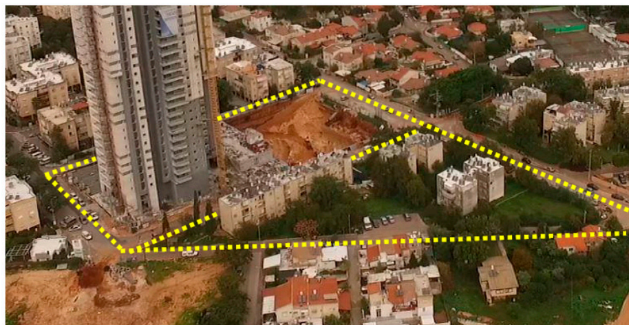
Figure 2. The first completed building (Local Planning Scheme No. PT/1238/16).
