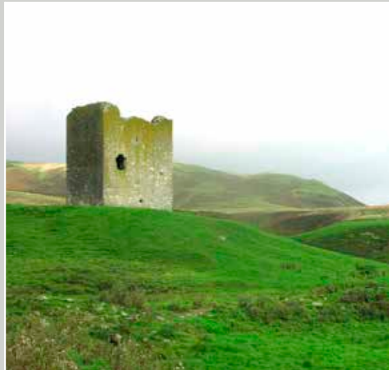
Dryhope Tower Scottish Borders Structural Repairs with Simpson & Brown, Architects
