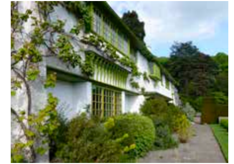
Garden façade, Perrycroft
