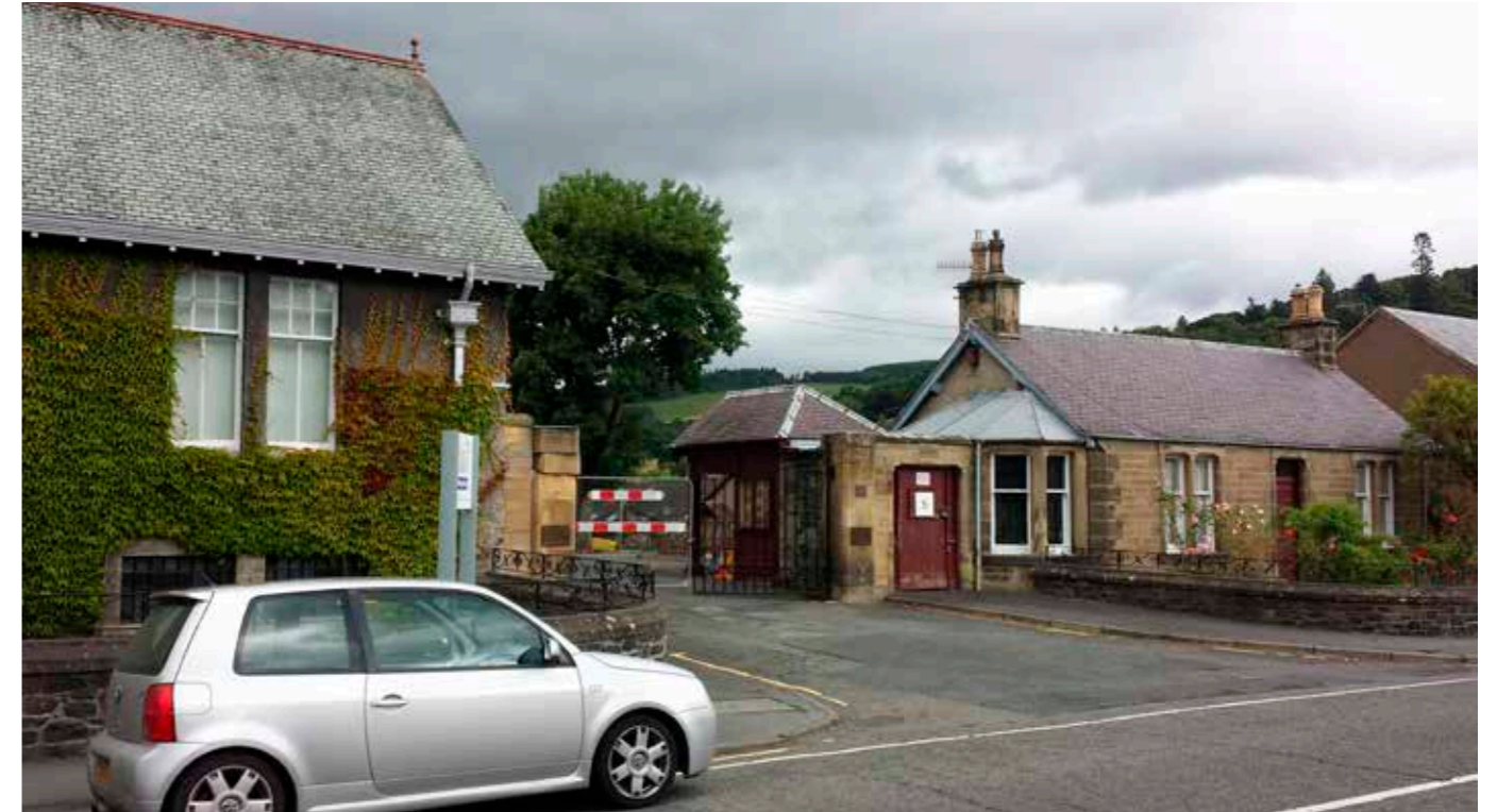
The main gateway at the Royal Infirmary site, Lauriston Place (Edinburgh) – the right-hand cottage, but not attached lodge/gate on the left, will be retained.
