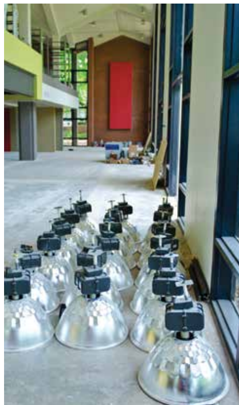
Major renovations continue in the Davis Memorial Library
