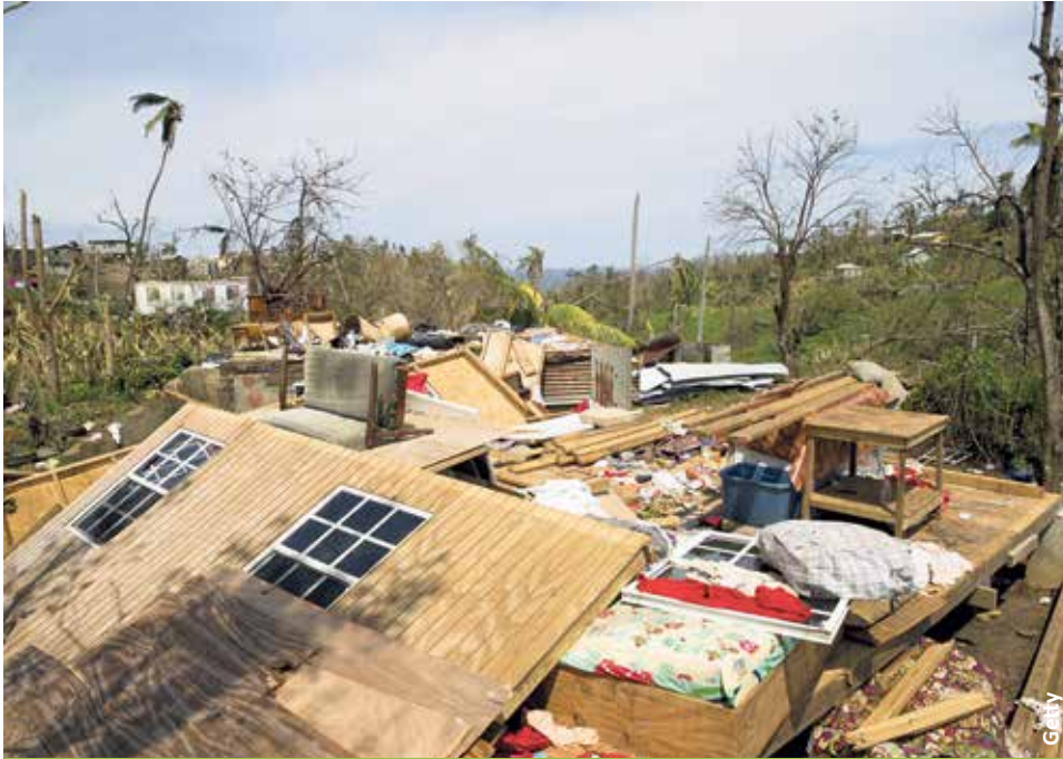
WESLEY, DOMINICA: A destroyed home after Hurricane Maria rampaged across the Caribbean island, killing dozens of people.
