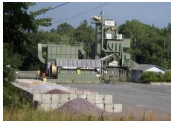
(asphalt batch plant)
