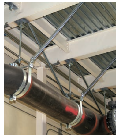
TOLCO seismic bracing
