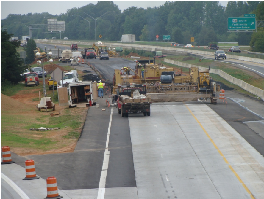
unbonded concrete “white topping” overlay
