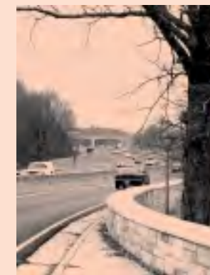
The Baltimore-Washington and Suitland parkways establish a precedent for urban highways, with landscaped medians and quality materials.
