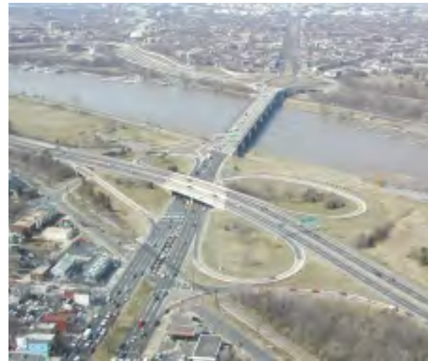
The site of the future Pennsylvania Avenue Gateway. Currently Washington's great avenues and the Anacostia freeway cross one another with complicated interchanges.
