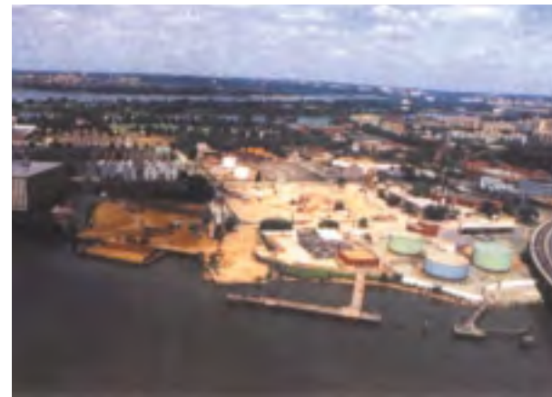
Oil storage facility immediately south of the Frederick Douglass Bridge.
