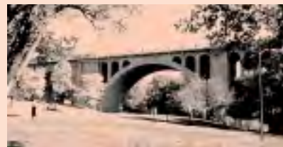
Taft Bridge in Rock Creek Park.
