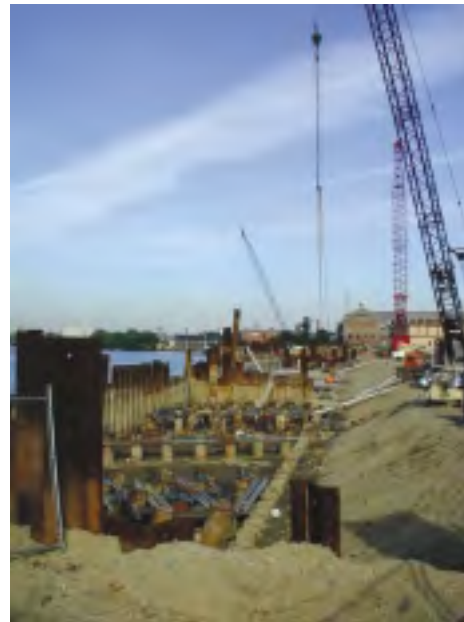
Recent construction at the Southeast Federal Center
