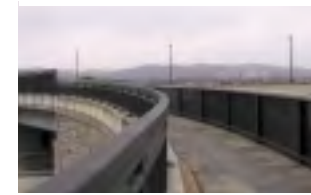
3 The pedestrian zone on the John Philip Sousa Bridge at Pennsylvania Avenue...
