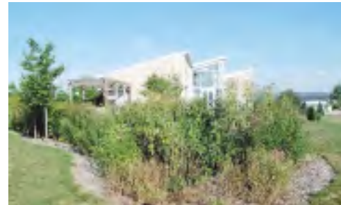
Two examples of how a bio-swale catches and filters rainwater around a building, while also functioning as a beautifully designed landscape.
