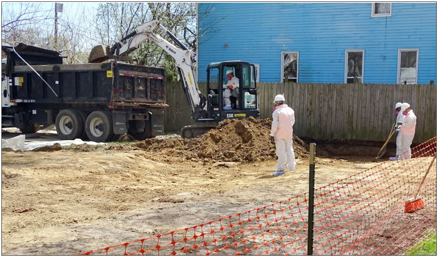
(Photos courtesy of USACE, Louisville District)
