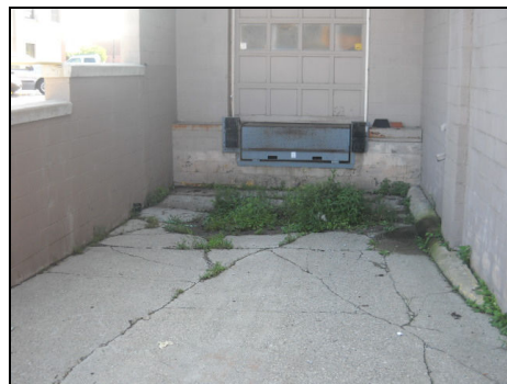
View of truck well.
