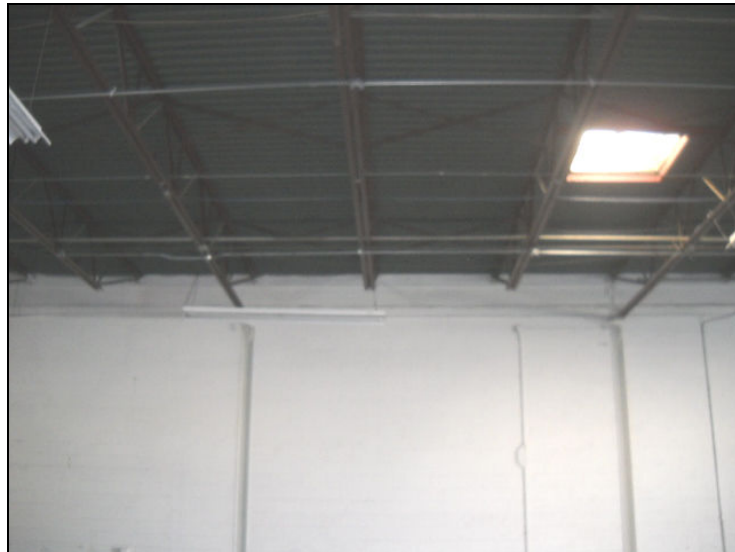
View of structural components and build methodology.
