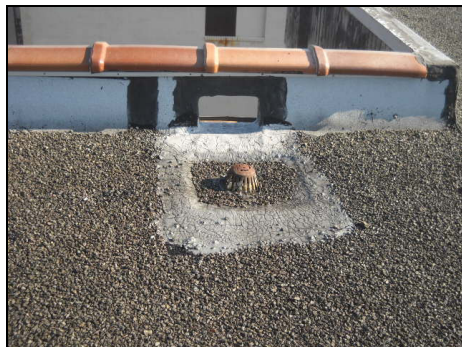
Roof drains need to be cleared of debris.
