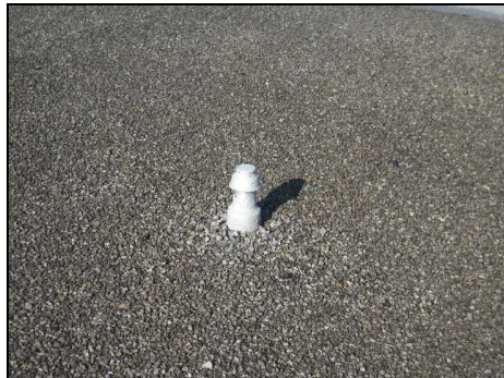
Roof well vented.
