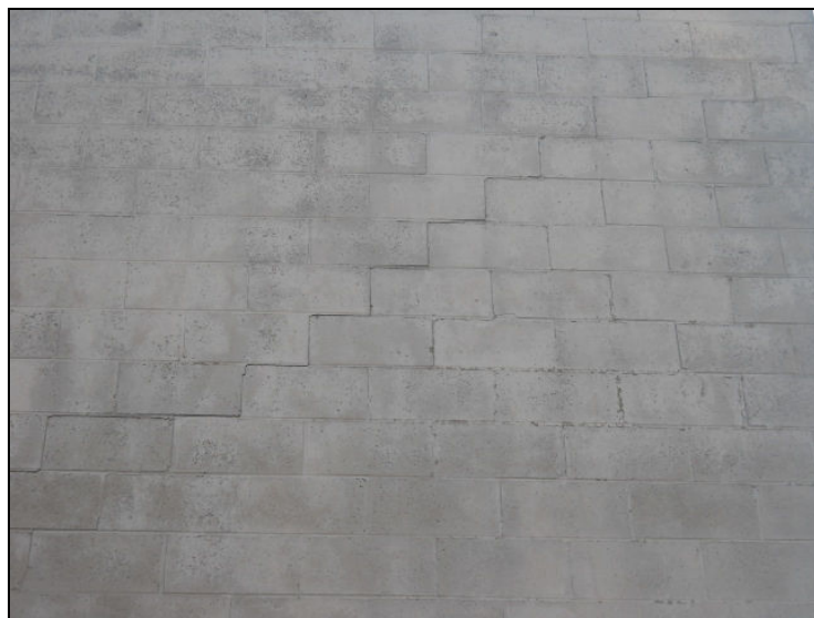
General condition of block exterior wall.
