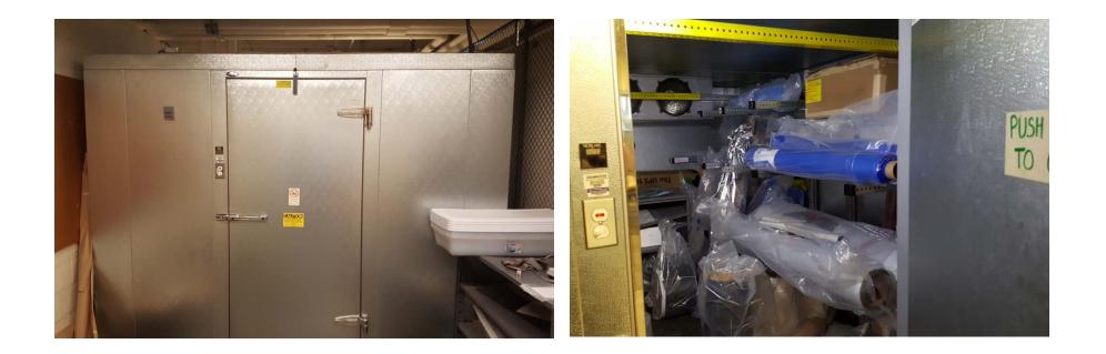
The ME Department walk-in freezer is used to store prepregs, thin-film adhesives, etc, and maintains a temperature of -18°C (0°F)
