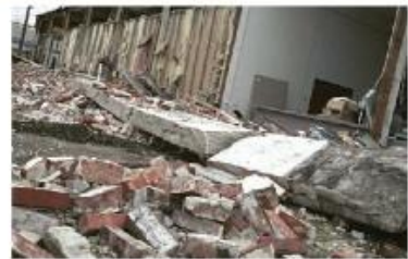
Earthquake damage in Washington in 2001
