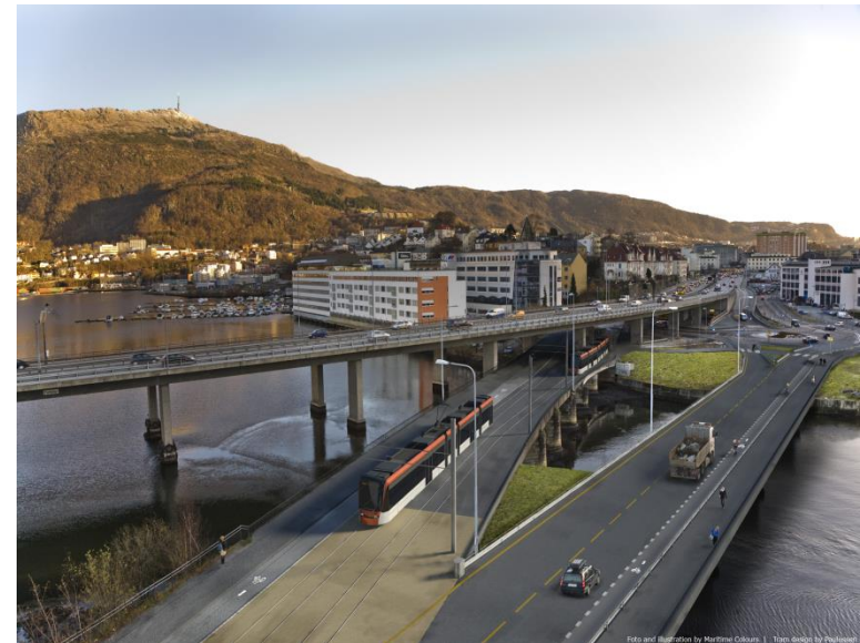
Bridge, Strømmen Norway
