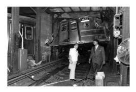
According to accident investigators, Ray had been running the train at 50 mph in a 10 mph zone and took the switch so fast that only the front of the first car made the crossover. The third and fourth cars ended up perpendicular to the tracks, shearing off support columns and split in half. The line suffered heavy damage, and service was disrupted for six days. The entire infrastructure, including signals, switches, track, roadbed, cabling, and 23 support columns, needed to be replaced.
