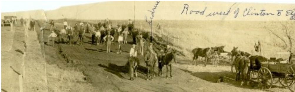
Much of Route 66 was originally built with horse or mule drawn road implements. This construction is west of Clinton, Oklahoma. Circa 1927.
