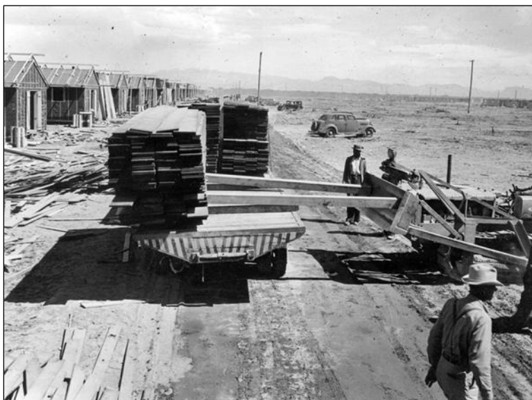
Lumber to be used in construction of barracks is being unloaded at Site I at the Colorado River Relocation Center (Poston).
