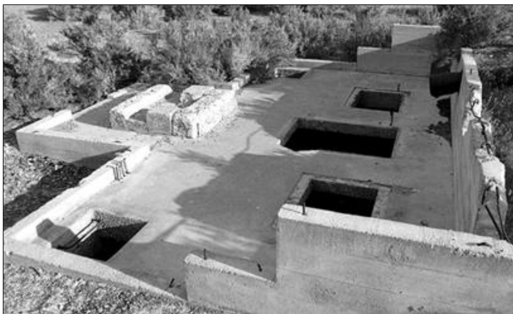
Foundations remain at the Topaz Relocation Center. National Park Service photo, 2002
