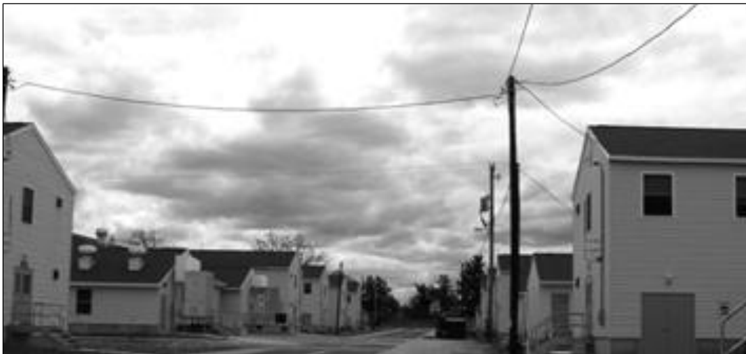
The barracks at Fort McCoy have been modernized and are still in use. National Park Service photo by Michele Curran, 2010
