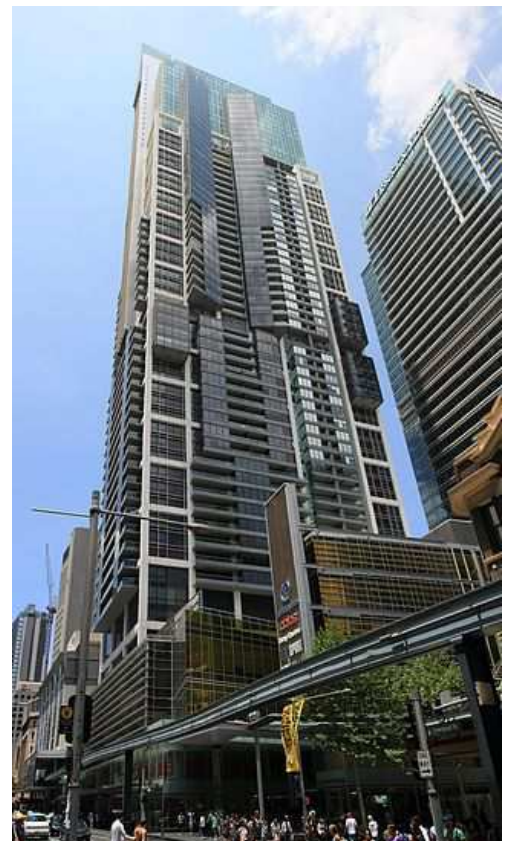
Above : The "Construction Site" is now known as "World Square" in the 21st Century. The famous Sydney Monorail, which features heavily in the third act - is now no more. It was decommissioned in 2014 and the track has now been removed.
