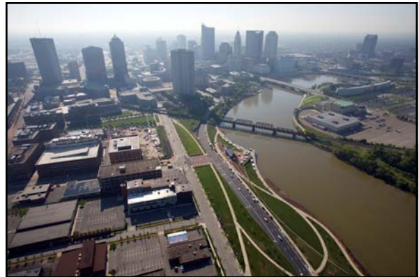
North Bank Park
