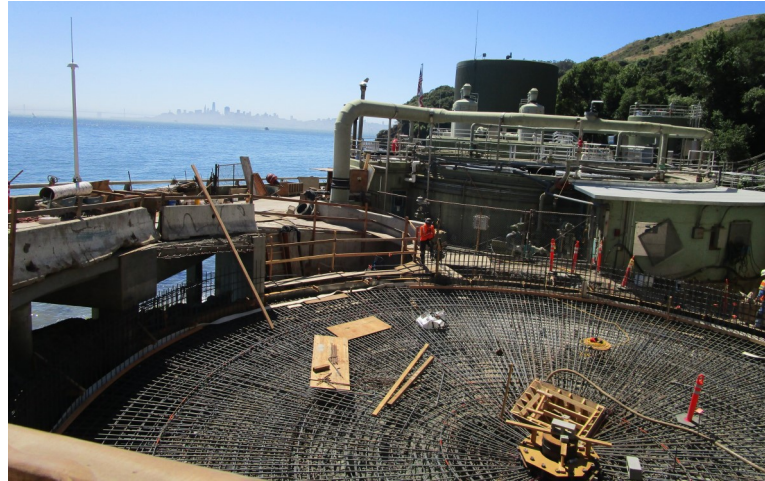
Primary Clarifier Designed by TJCAA—Currently under Construction in the San Francisco Bay Area
