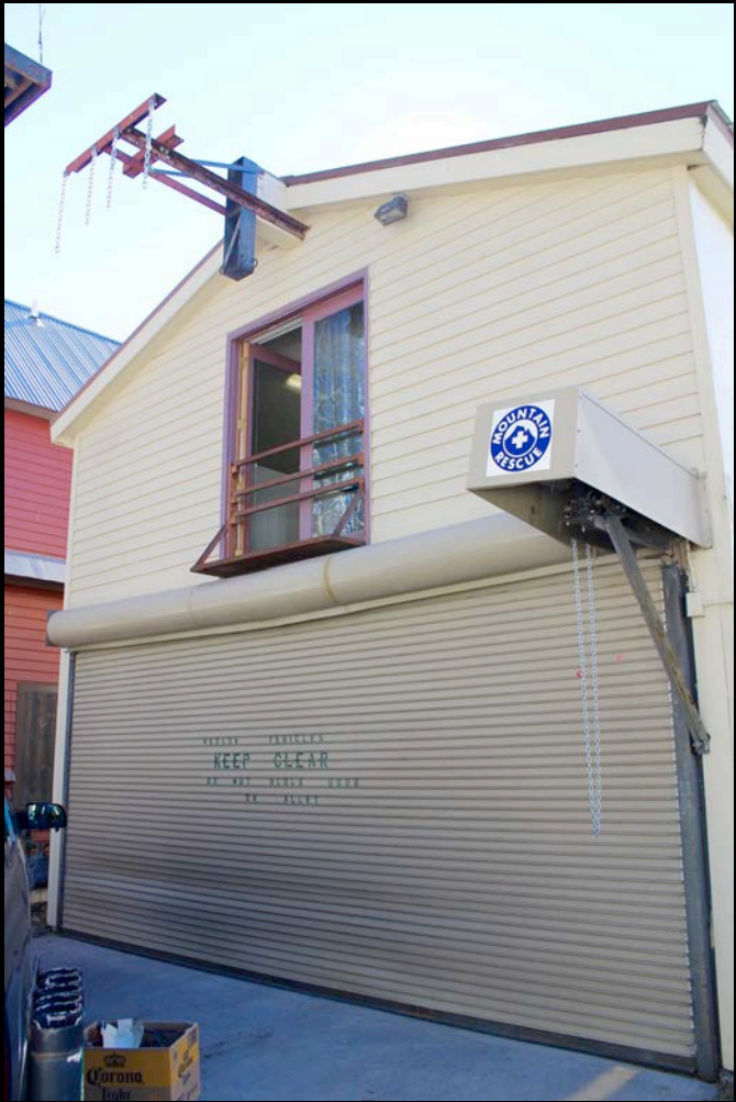
North (rear) Wall of the Building View to the Southeast
