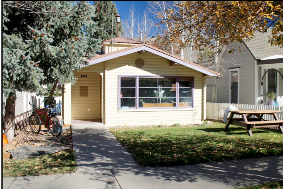
View of the Property from Main Street View to the North
