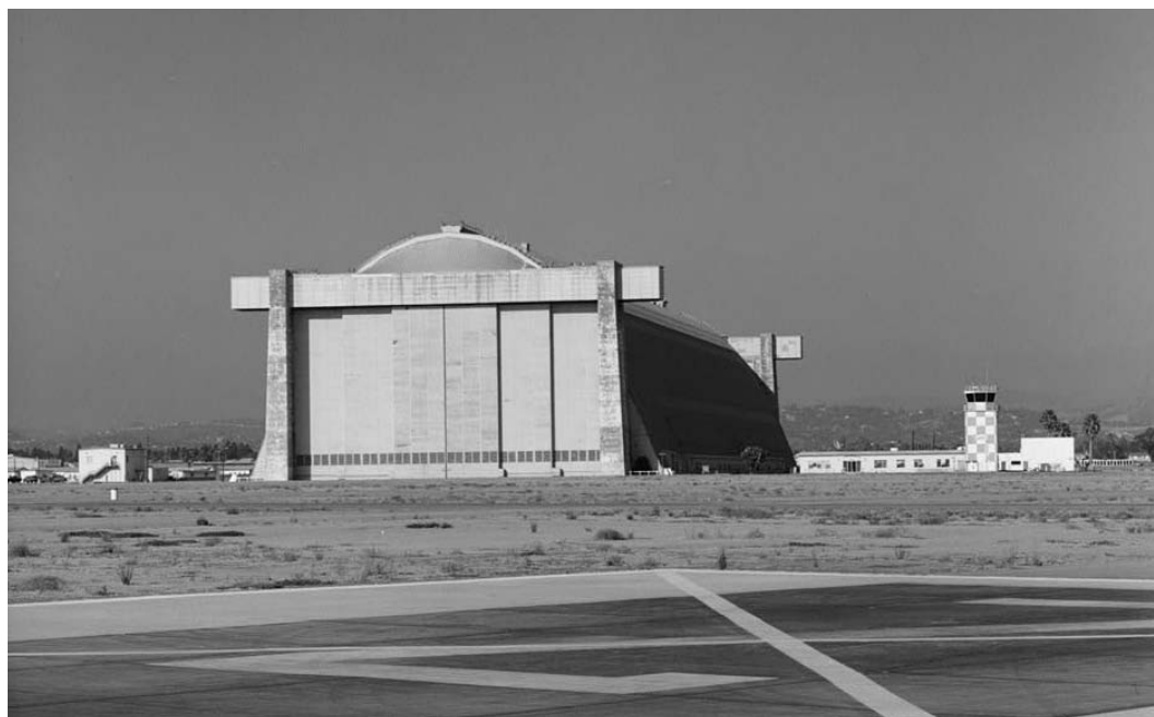
Building 28, south view, control tower on right, 1999
