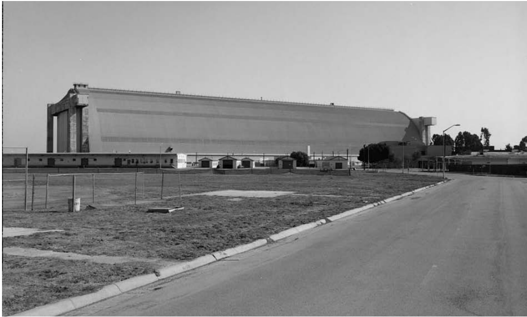
Building 28, west side, 1999
