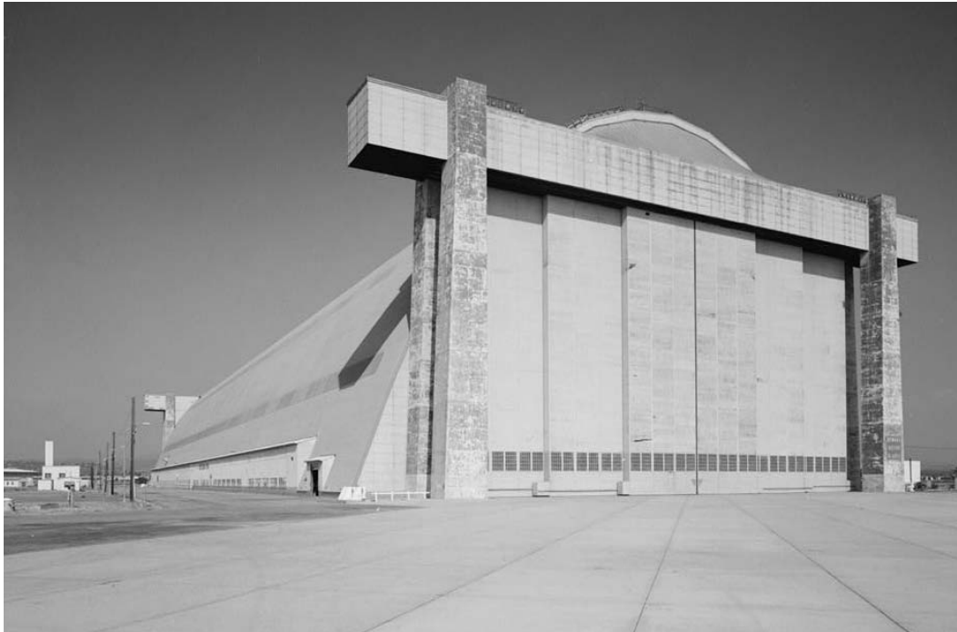
Building 28 (Hangar 1), south doors, 1999
