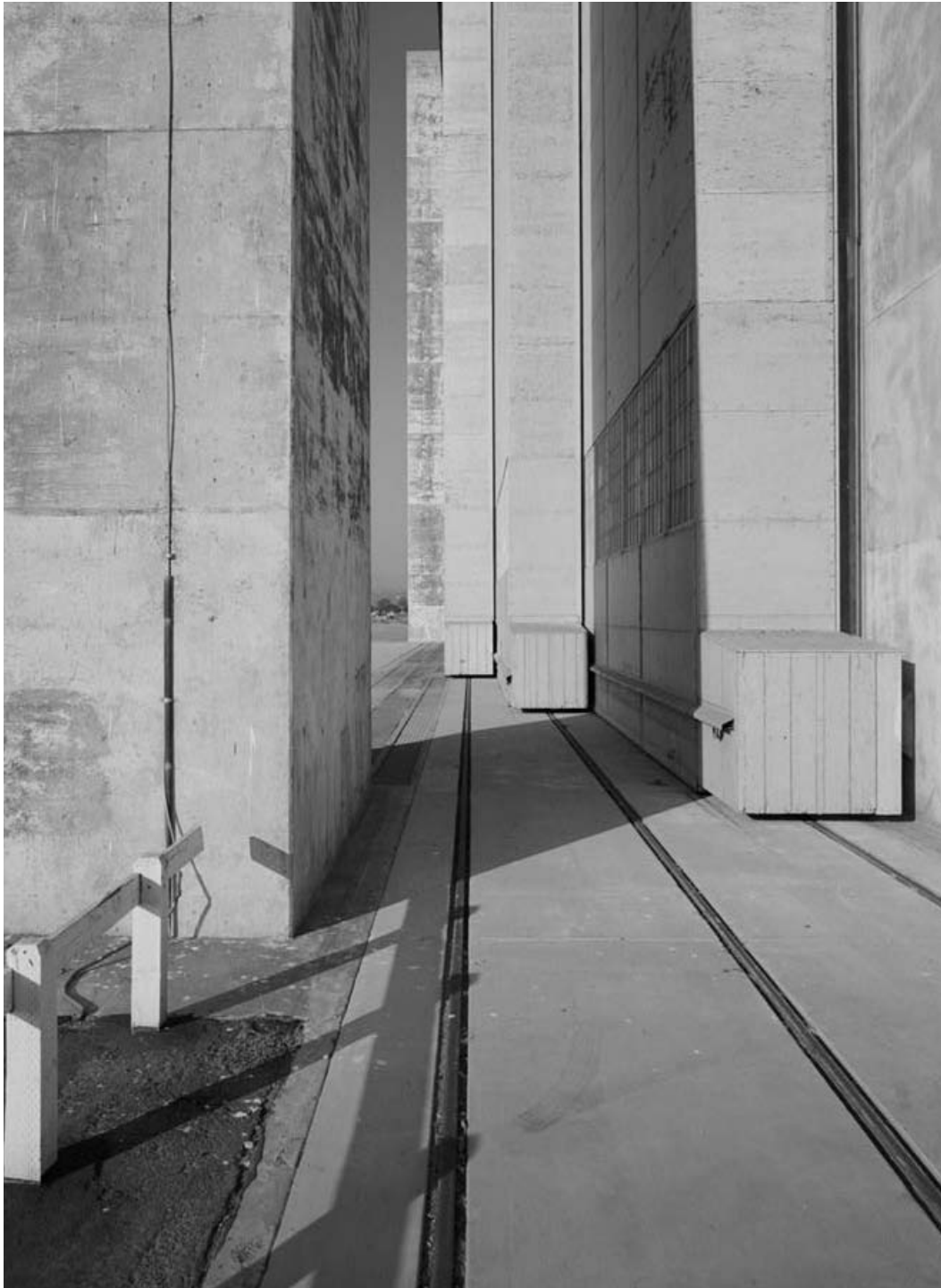
Building 29, west doors, on rails, 1999
