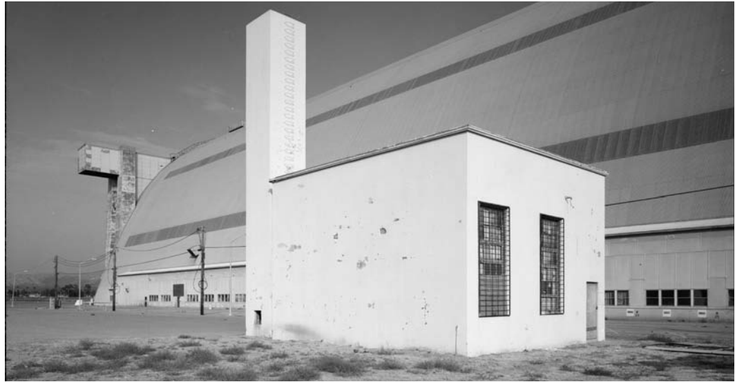
Helium Tank Building No. 1 (Building 28A)
