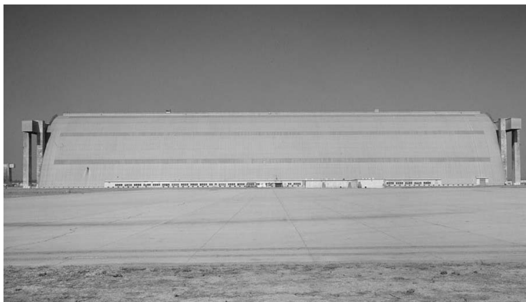
Building 29, side view, 1999
