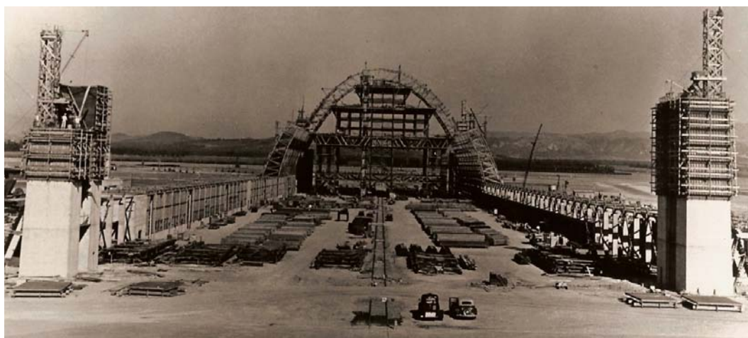
Hangar under construction, 1942
