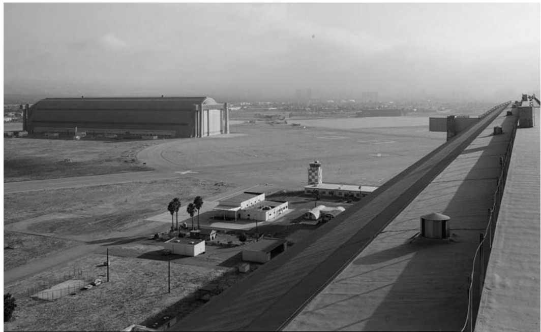
Building 29 on left, viewed from roof of Building 28, 1999
