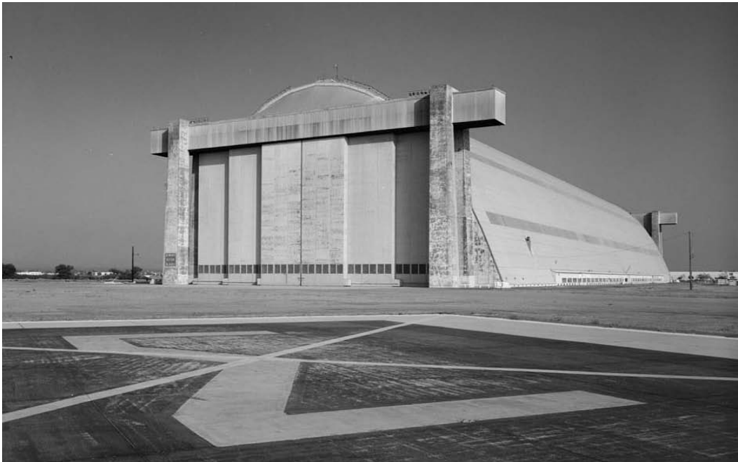
Building 29, west doors, 1999
