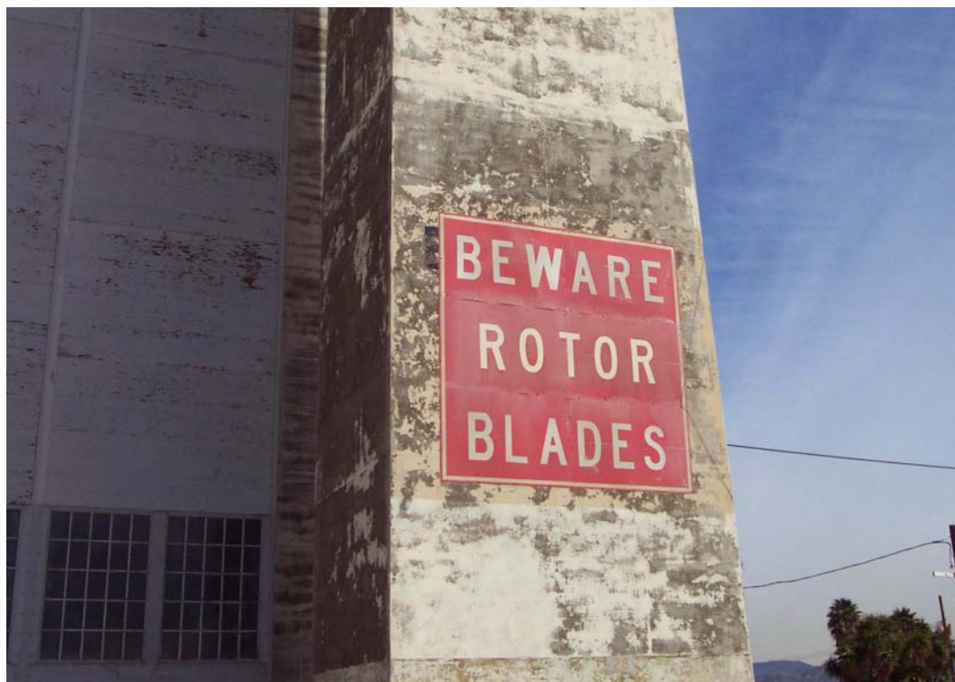
Warning sign, Building 28, March 2002
