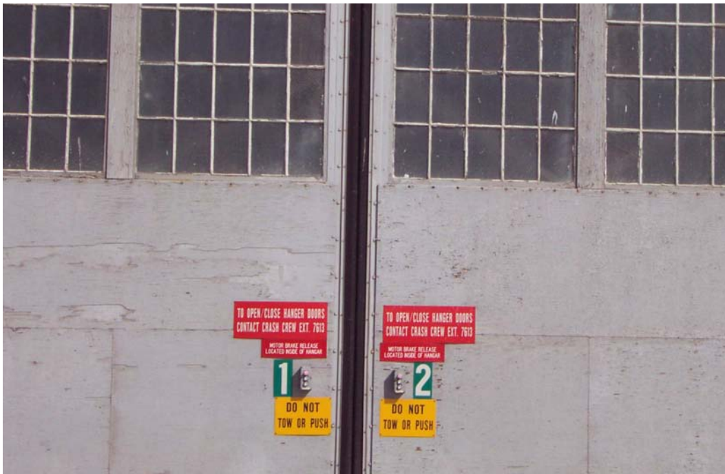
Building 28 exterior, south door detail, March 2002
