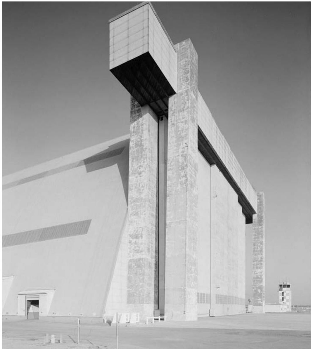
Building 28, south doors, 1999
