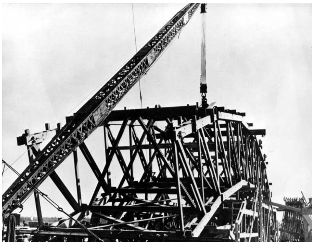
Hangar roof truss being set in place, 1943
