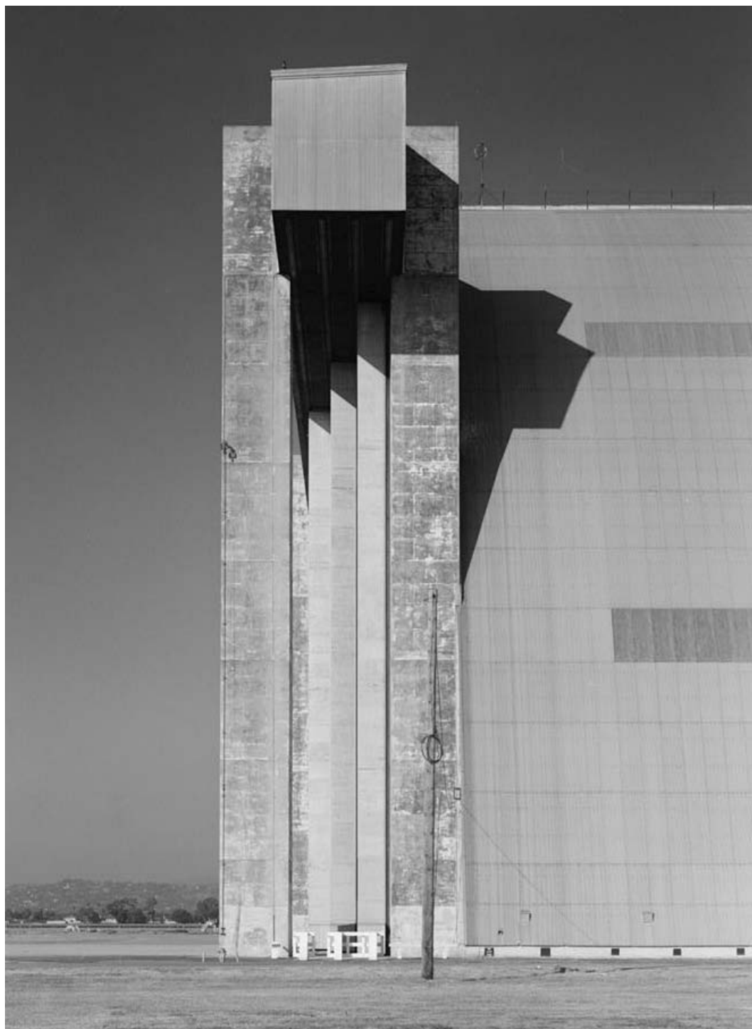
Building 29, west doors, 1999
